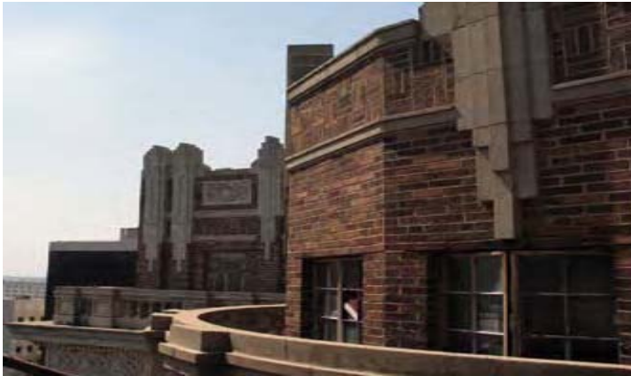
Figure 2.13: Historical Brick Building under Renovation.
