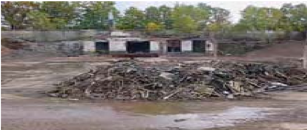
Figure 2.10: Debris from Trees, Brushes and Soil Removed During Site Clearing. Source: (EPA, 2009B).
