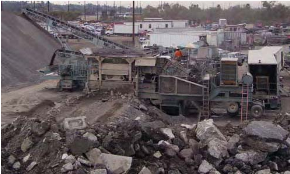
Figure 2.6: Asphalt Paving Recycling Site. Source: (EPA, 2009B).
