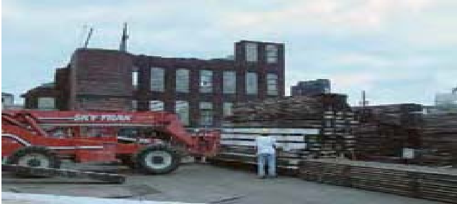
Figure 2.7: Different Sizes of wood Arranged at building Deconstruction Site. Source: (EPA, 2009B).
