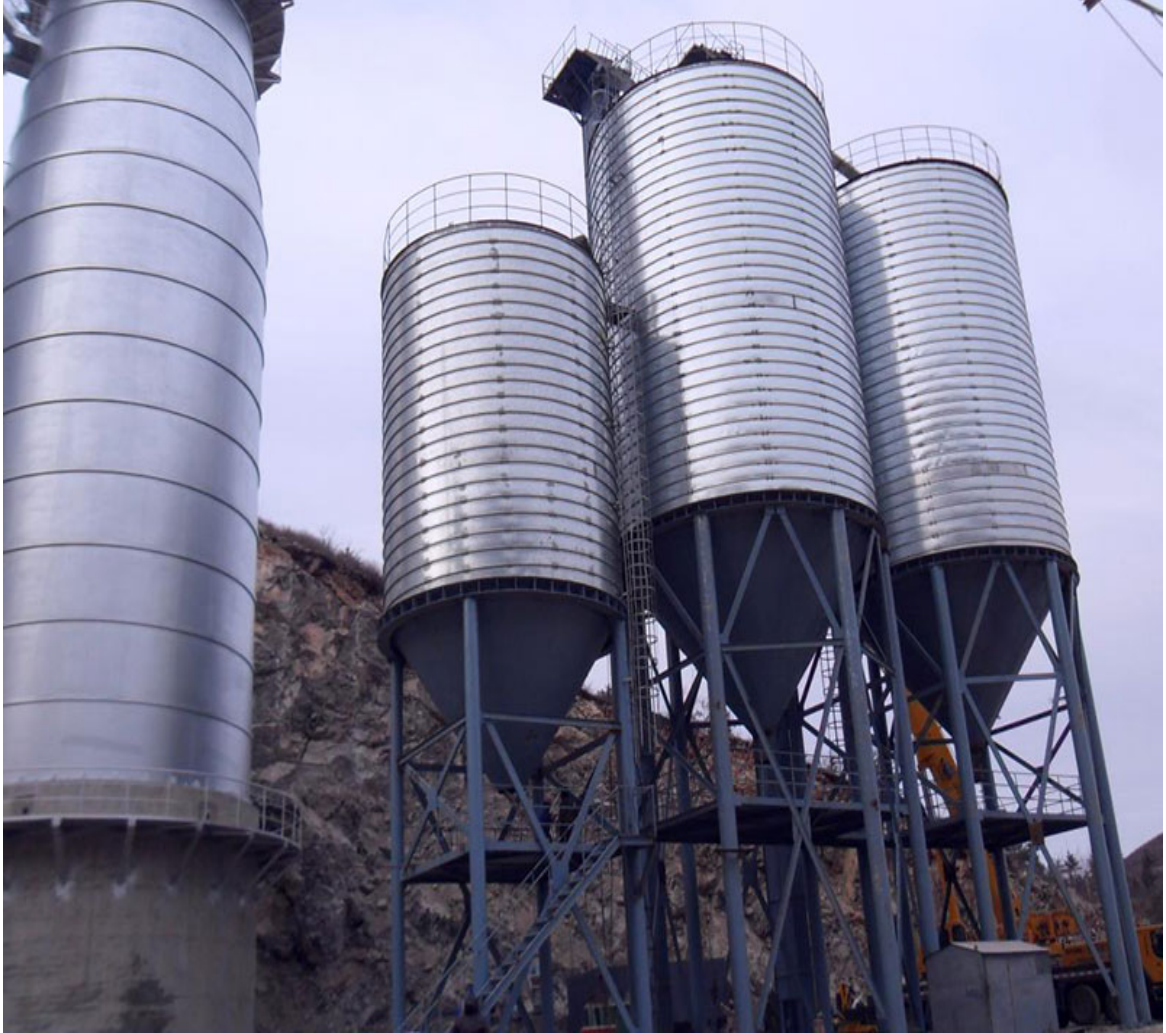
Figure 2-4: A fly ash silo at the plant
