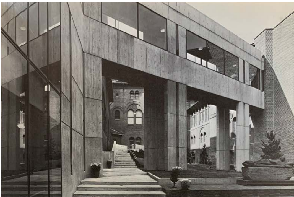
Figure 7: The diagonal bridge which spans the courtyard, connecting the old museum to the new addition.
