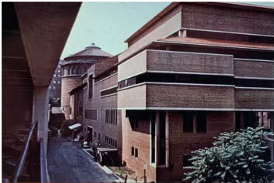
Figure 4: Exterior of the addition showing the connection with the original museum's rotunda in the rear.
