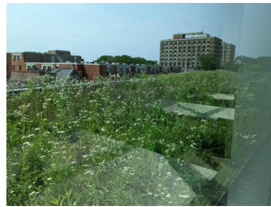
This view of the Charles Library green roof illustrates how a field of plants radically transforms what is otherwise a drab urban landscape
